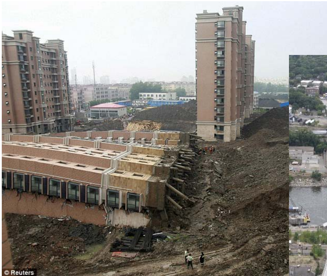
Residential Tower Shanghai, 2009
